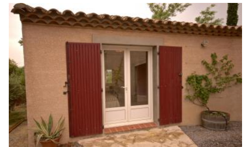
Front entrance and Parking
