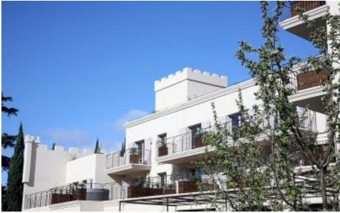
An outside view of the apartments in The Distillerie.
