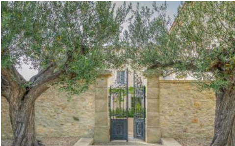
Gates to courtyard
