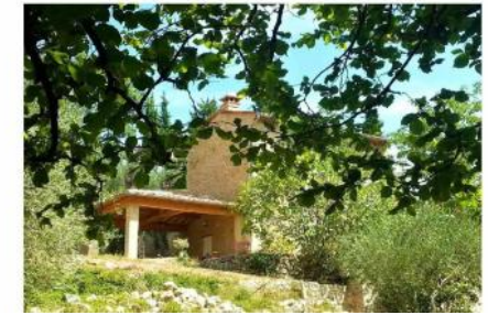
South west side
