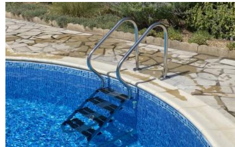
New "comfort" pool steps added 2024
